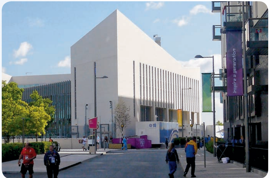
The Polyclinic, located in the Athletes' Village in Olympic Park, was home to a Discovery MR750w 3.0T and an Optima MR450w 1.5T with the GEM Suite of coils. The MR systems were housed inside the trailers.
